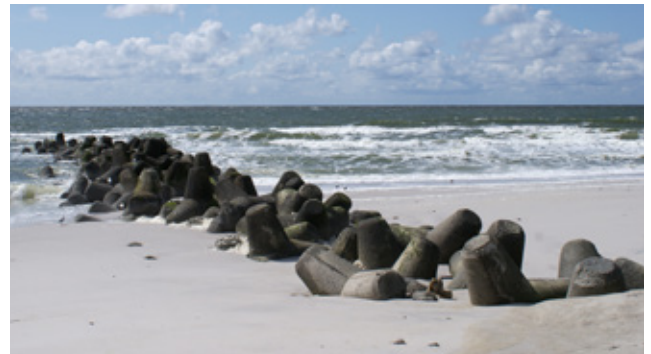
Tetrapodes for coastal protection near Hörnum on the island of Sylt, German North Sea Coast
